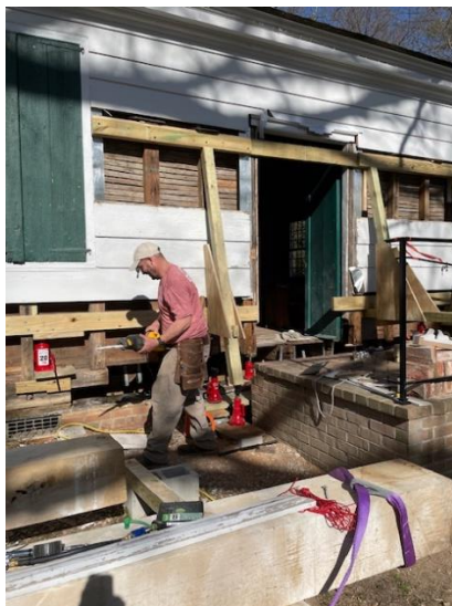
David Weir and John O'Rourke in the sill replacement process.
