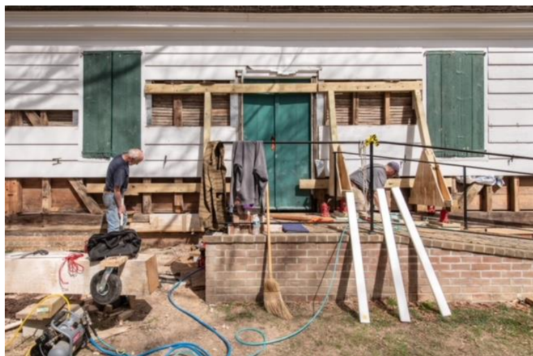
David Weir and John O'Rourke in the sill replacement process.
